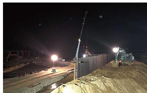
Photo 2.4 Completion status of steel sheet pile double cofferdam<sup>18)</sup>
