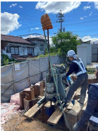
Fig. 3. Insertion of injection pipe
