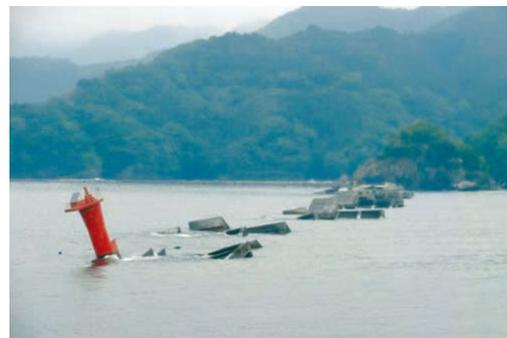
Photo 1.10 Damage to Kamaishi Bay mouth breakwater<sup>10)</sup>
