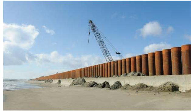
Photo 1.12 Installation of tubular sheet piles on the Higashihama coastal embankment of Ishinomaki Port<sup>14)</sup>
