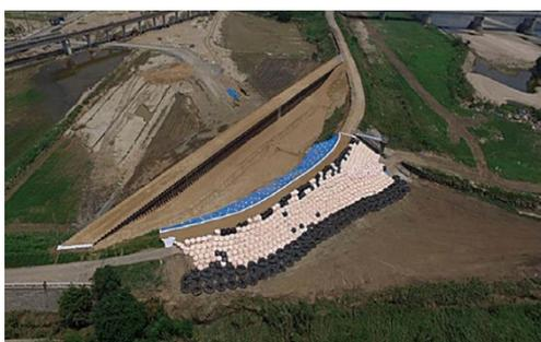
Photo 2.3 Double cofferdam of steel sheet piles driven 24 hours a day<sup>18)</sup>
