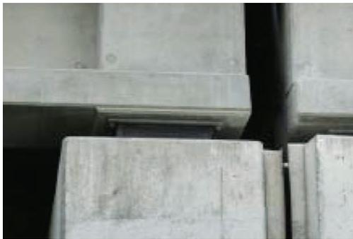
Photo 1.9 Bearing deformation<sup>11)</sup>
