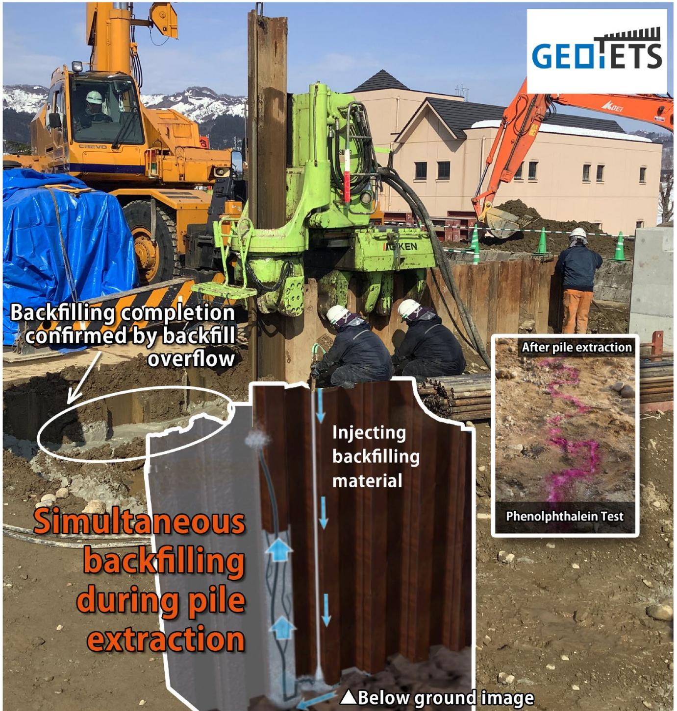
Fig. 1 Overview of GEOTETS Method
